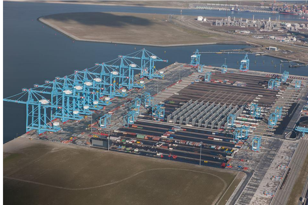
APM Terminal – Rotterdam port
